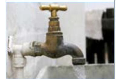
Taps installed in various campus locations
